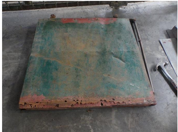
Image 24 (a&b). It is important to undertake regular maintenance on metal structure and sliding doors, before it represent a risk to break or injure animals and staff.
