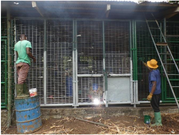
Image 26 (a&b). Construction workers Richard NDANJI and Kum FERNANDEZ applying the first layer of anti-corrosion paint on Western lowland gorilla Chella night den. Team work allows for faster progress and limits the days when the gorillas cannot go out.
