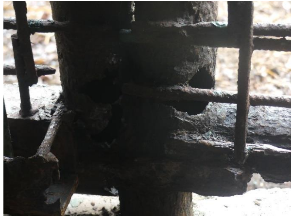
Image 23 (a&b). View of some damaged pipe in Western lowland gorilla Chella night den. The salty sea breeze and constant humidity are strong degrading factors for all the metal structures.
