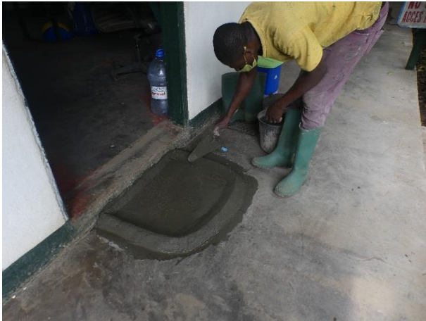
Image 19. Construction worker Richard NDANJI creating a footbath at the main entrance of the vet clinic.
