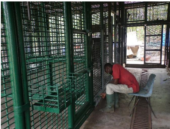
Image 28 (a&b). Construction worker Jacob TEBO applies the second layer of anti-rusting painting as a finishing touch for Western lowland gorilla Chella night den.
