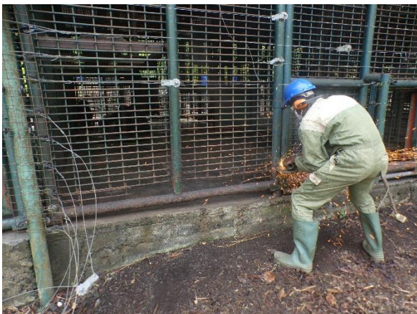
Image 25 (a&b). Construction worker Leonard GEH is cutting off damaged metal pipe and rod in front of Western lowland gorilla Chella night den to replace them.
