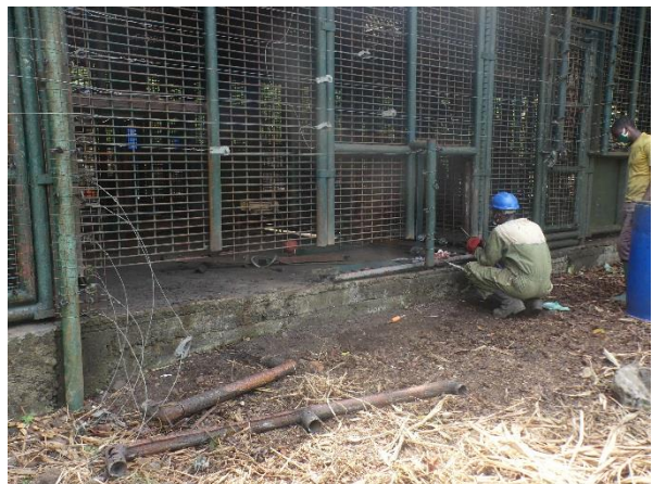
Image 25 (a&b). Construction worker Leonard GEH is cutting off damaged metal pipe and rod in front of Western lowland gorilla Chella night den to replace them.
