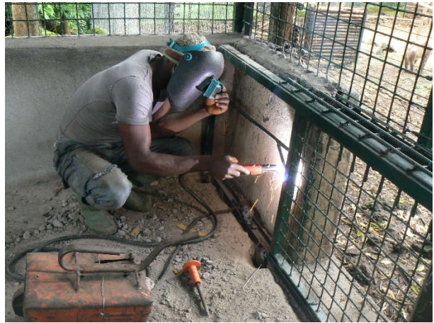
Image 22. Replacement of door rail and door maintenance (upper Drill satellite cage).
