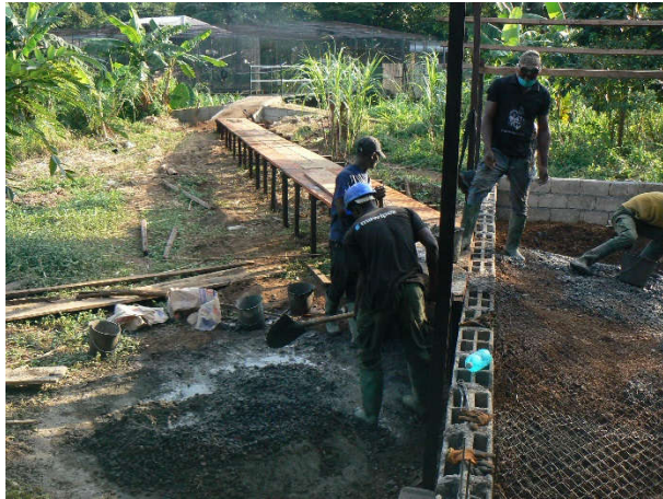
Image 17. Side view of install wooden path.
