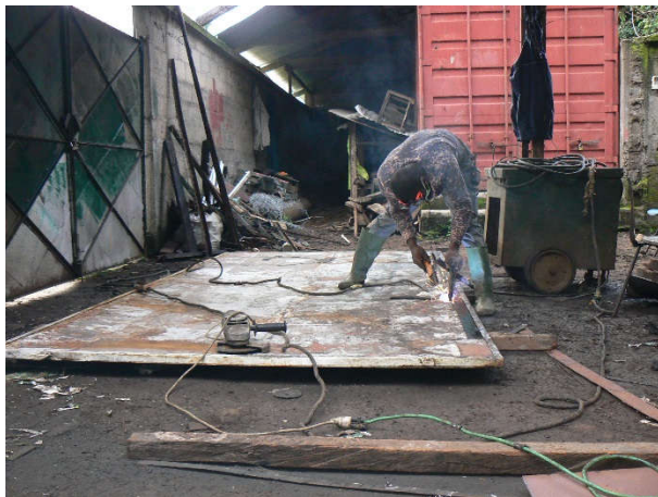
Image 29. Welding work of some damage area in the billboards.
