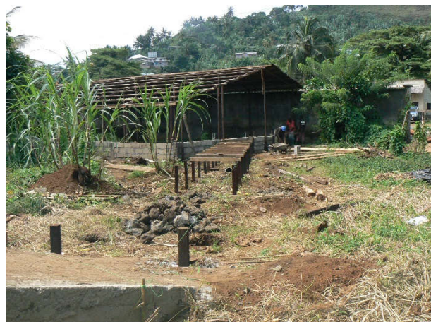
Image 14. Elevated wooden path installation.
