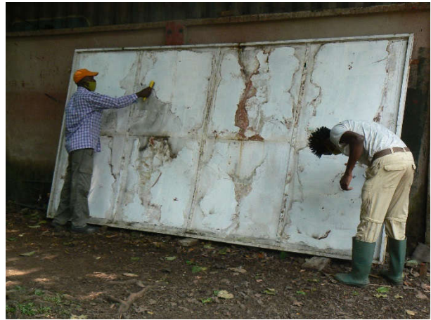
Image 28. Cleaning and wire brushing.
