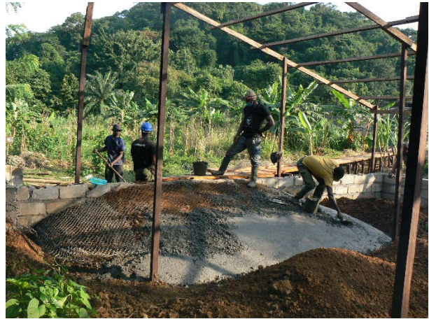
Image 16. Ramp concreting.
