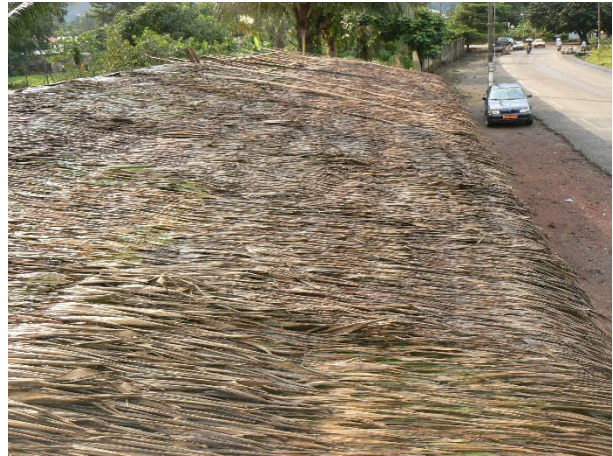
Image 18. Continuation of traditional Raphia palm mat roofing.
