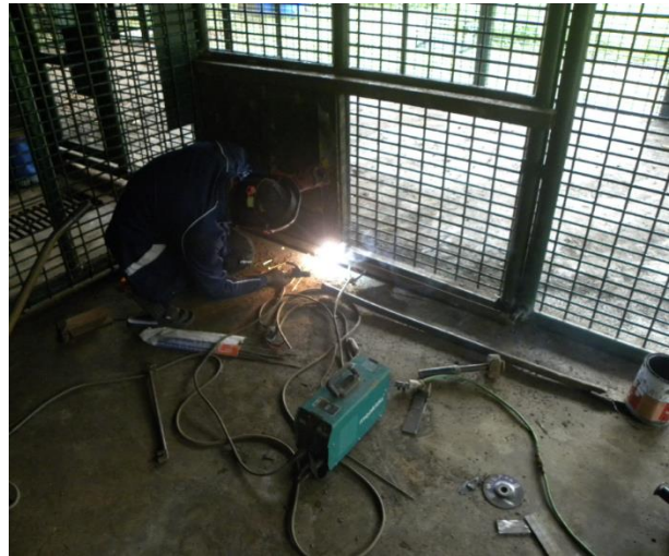
Image 21. Our expert construction team can weld and install everything themselves
