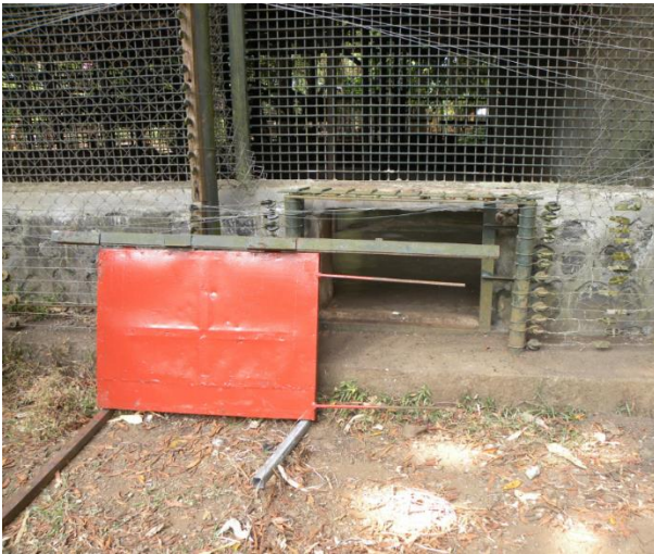
Image 20. Old and rusted parts of the night dens had to be cut away and replaced
