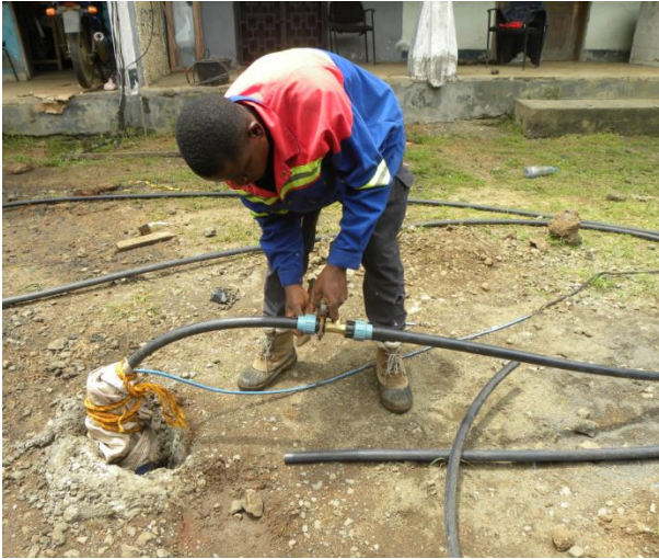
Image 18. The new borehole has been completed and connected to the existing pipes at the LWC
