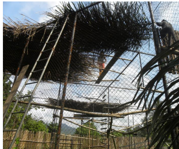
Image 29. To protect our guenons during the dry season we installed additional shades made from dry palm leaves to help them hide from the strong sun
