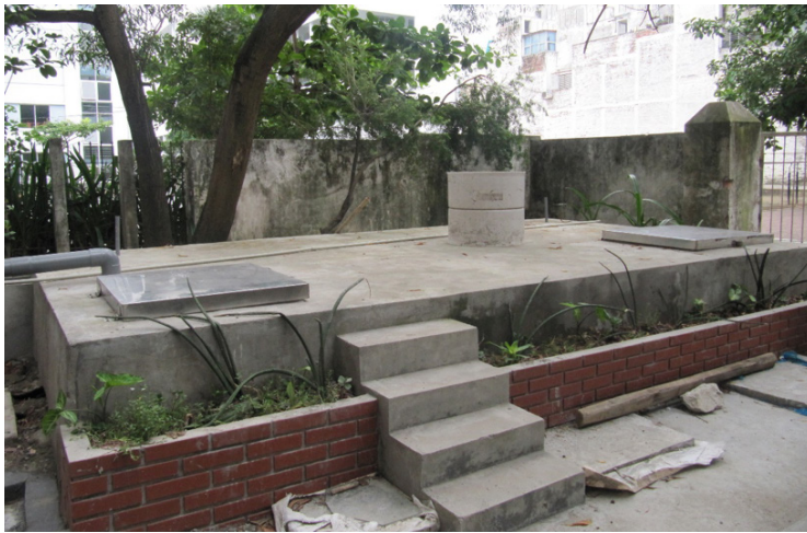
Drainage system improvement (Pathway-Receptor control). Source: Nguyen Viet Anh et al. 2020 "Policies study on rainwater harvesting for drinking in Vietnam" – final report for WASAT
