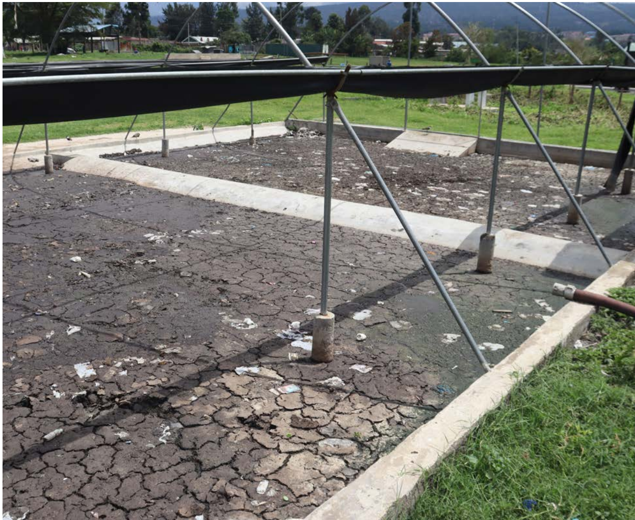
Old town faecal sludge treatment plant, Nakuru, Kenya © NAWASSCO
