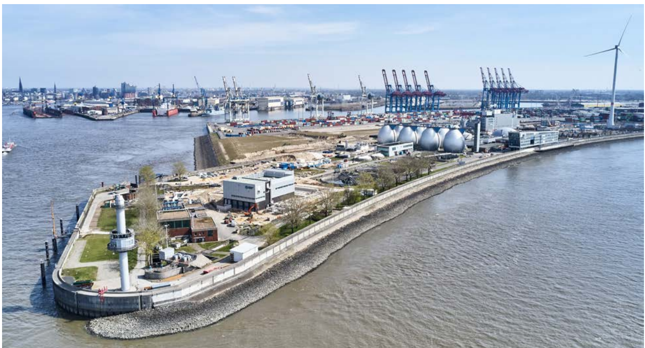
View of Hamburg waste water treatment plant © Hamburg Wasser
