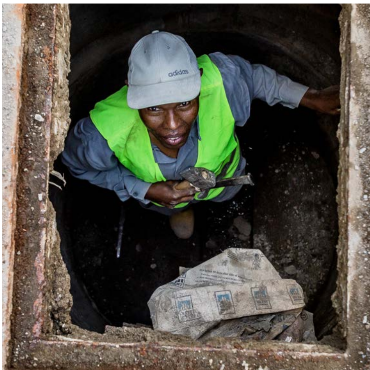
Worker inside sewer tank, Nakuru, Kenya © Brian Otieno
