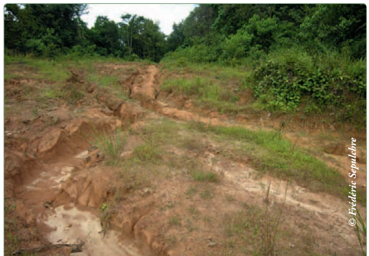
Photo 2.7: The erosion settles gradually on the abandoned logging roads
