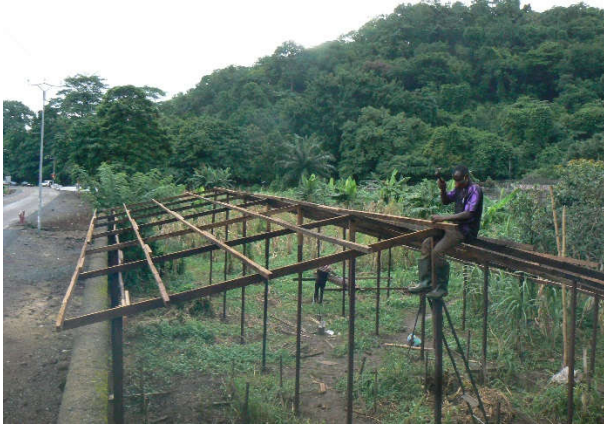
Image 26. Roof installation to provide shared to the composting area.
