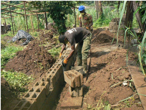
Image 28. Concreting and building of block wall to protect the composting area.
