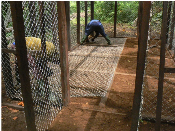
Image 20. Wire mesh installation on the ground floor panel.
