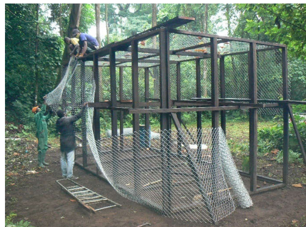
Image 19. Wire mesh installation on the soft-release aviary.
