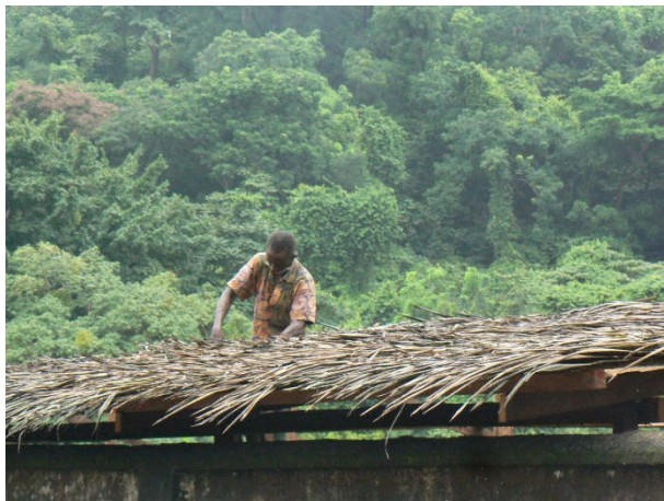
Image 32. Caleb Ngombe, from Mukunda village, is one of the rare experts to make traditional Raphia palm mats in the region. He also masters how to place them to ensure impermeability of the roof. In the past months, we have extended the number of palm mats: it is more natural and eco-friendlier, does not heat like zinc sheet and make less noise when rain falls, hence providing a more comfortable shelter to animals. Unfortunately, because of modernity, this expertise is threatened and we aim to boost the activity to support Caleb but also encourage the youth to conserve this beautiful and useful expertise.
