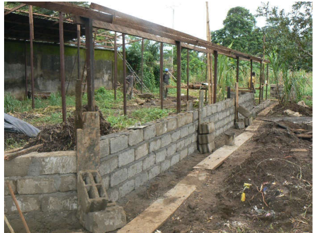
Image 29. Concreting and building of block wall to protect the composting area.
